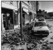
Downtown Santa Cruz was severely damaged by the 6.9-magnitude Loma Prieta earthquake in October 1989. Steve Castillo/The Chronicle
